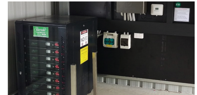
Rack-mounted lithium battery
